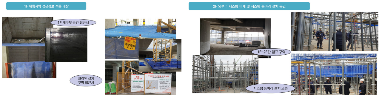
Fig. 2. Example of scaffolding and hazardous area empirical site
